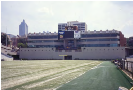
Figure 91 - William C. Wardlaw, Jr. Center. Georgia Tech Facilities Department Photographs and Slides
