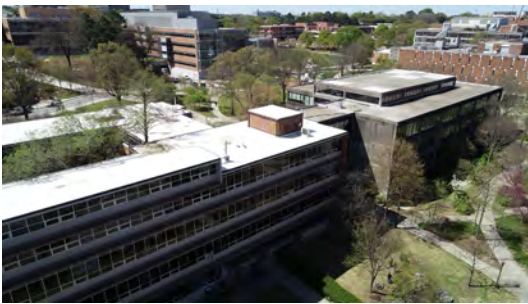
Figure 109 - Aerial image of Architecture East (foreground) and Architecture West (background).
