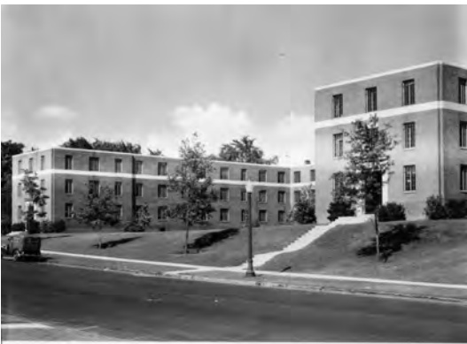
Figure 63 - Techwood Dormitory. Georgia Tech Photograph Collection
