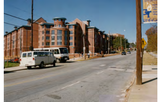
Figure 93 - Construction and preparation of Olympic Village housing. Georgia Tech Photograph Collection
