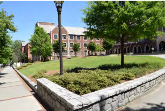
Figure 100 - Brittain Dining Hall Retaining Wall
